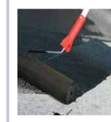
application of APP waterproofing membrane can be applied as a protective paint to
