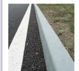
Concrete channels are important to keep the paving blocks intact, as it acts as a support for the paving blocks for a firmer fix and
