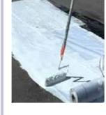
Marglass Mesh is essential to reinforcing the External Insulating Finish System. It can provide the system with enough capacity to contain the movements, caused by thermal excursions or shrinkage, or the insulating material over time, preventing the formation of hairline cracks on the facade.
