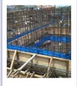
Water bar when embedded in the concrete ioints, acts as a continuous watertight diaphragm to prevent any seepage of liquids in constructions joints which are subject to hydrostatic pressure. It is designed for expansion or contraction joint, meanwhile, it can accommodate lateral and transverse movements which make it capable to suit the moving joints.
