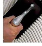
Creamy acrylic based compound specifically designed to bond flexible tiles to concrete and wooden surfaces. It may also be used for bonding wooden, parquets to floors, expanded polysterene ceilings and walls. Fibreglass insulations to walls
