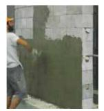
The application of thermablocks in internal dividing walls or partition walls.
