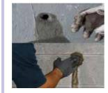
1. Hyseal 505 is an instant water plugging compound to stop water leakages
