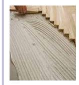
Polyflex Wood glue is a thick creamy based compound specially designed to bond wood,
