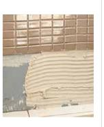
Polyflex Ceramic tile adhesive is a thick creamy based compound specially designed to bond Ceramic tiles to concrete surfaces
