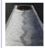
The shallow drain is used for storm water drainage for shallow water drainage where vehicles can pass over it and is used on the road itself or going across the road.
