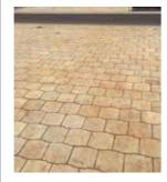
Concrete Interlocking tiles are mainly used for human traffic and also to protect the waterproofing layer underneath the tiles. Very famously used on where there are
