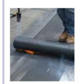
A gas torch is a vital tool in laying a proper App roof. Properly applied, the torch allows the roof to be completely sealed, making for a cost effective and durable roof. It's a skilled process, and involves playing with a lot of heat. We strongly recommend hiring a professional rather than doing this yourself if you make a mistake the risk of hurting yourself or severely damaging your property are extremely high.
